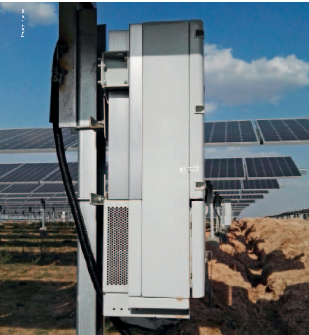
China's Huawei has been a pioneer in using string inverters in large-scale solar installations, developing plants in Germany and other parts of Europe, and is currently working on a 2 GW site in China.
